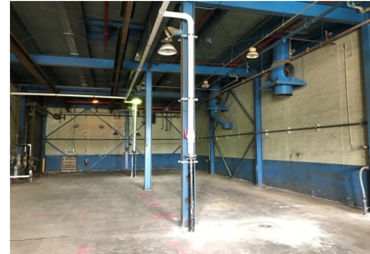
Industrial building with active vapor mitigation system
