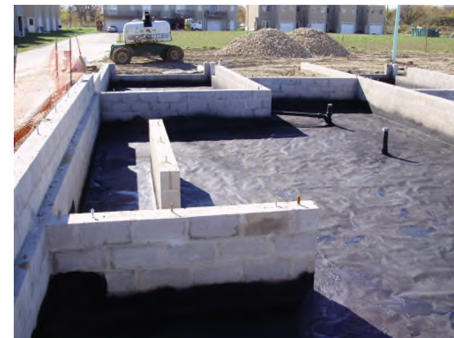
Example of a passive vapor barrier
